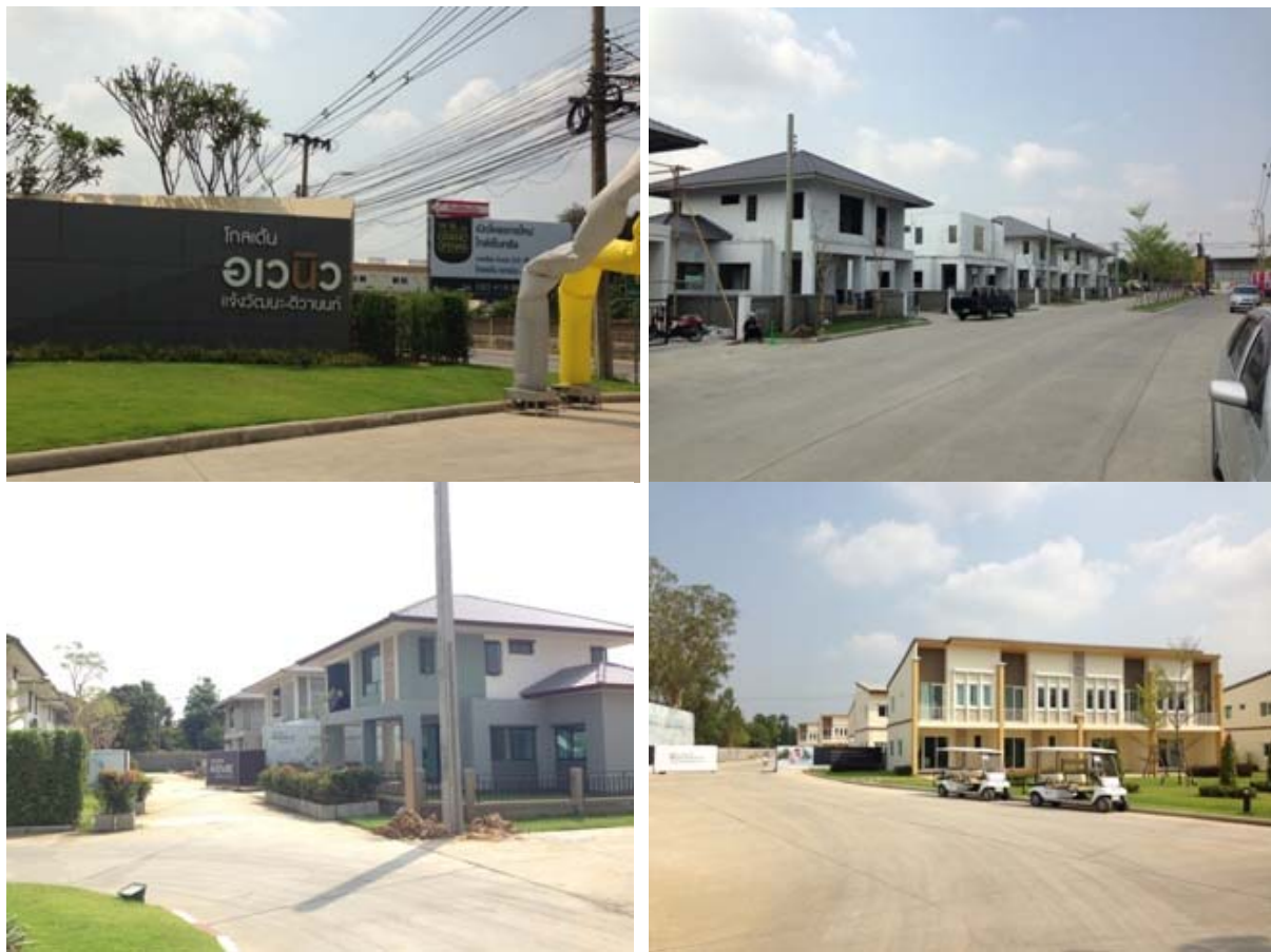
Figure 1 – 4: Photos of Golden Avenue Project, Tiwanon Road
